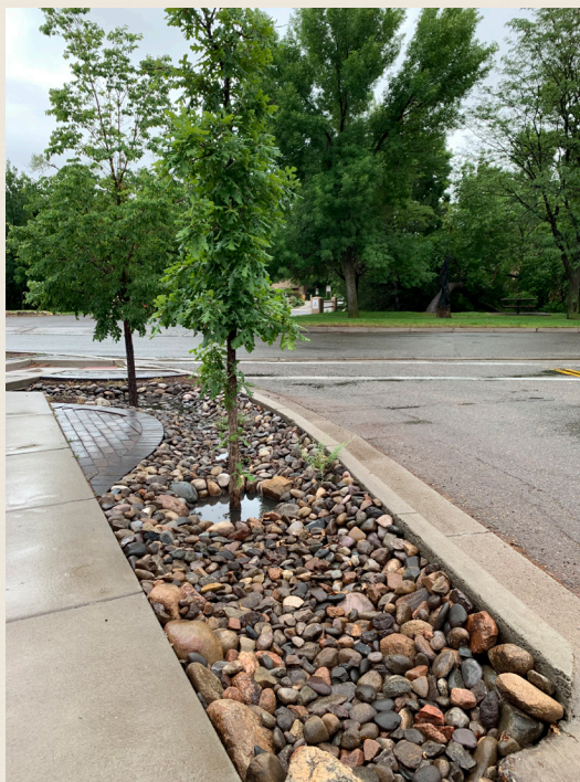
Above: A sediment trap, hidden under these river rocks and integrated into the design of this rain garden, helps filter stormwater and runoff to provide these trees with moisture that is essential to their survival and growth.
